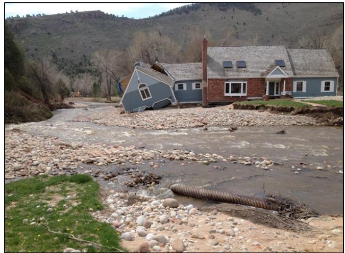
Avulsion on North St. Vrain Creek near Lyons, Colorado, through a residence during the September 2013 floods. Photo Credit: Michael Blazewicz (2013)
