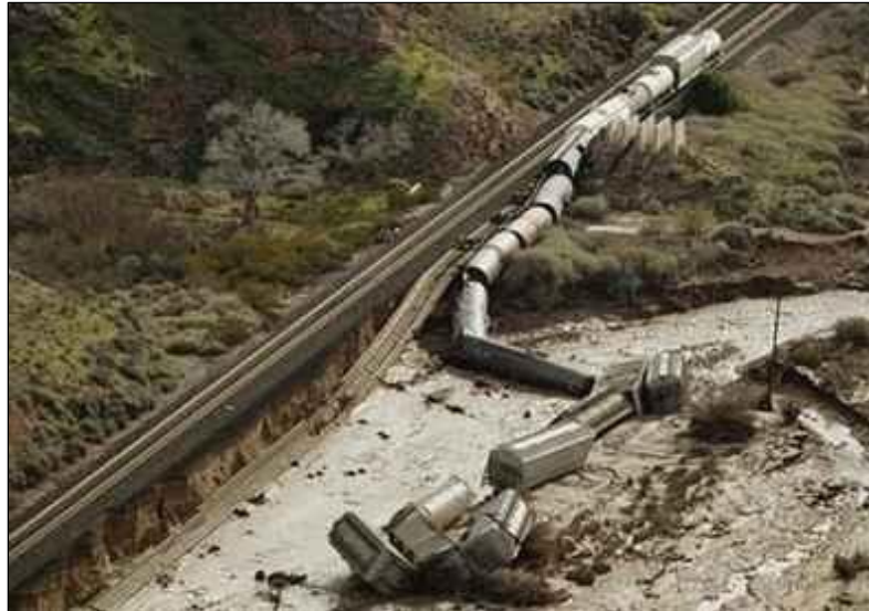
Photo caption: Caliente, Nevada. Train derailment caused by lateral erosion at the interface between a stream and adjacent transportation infrastructure.
